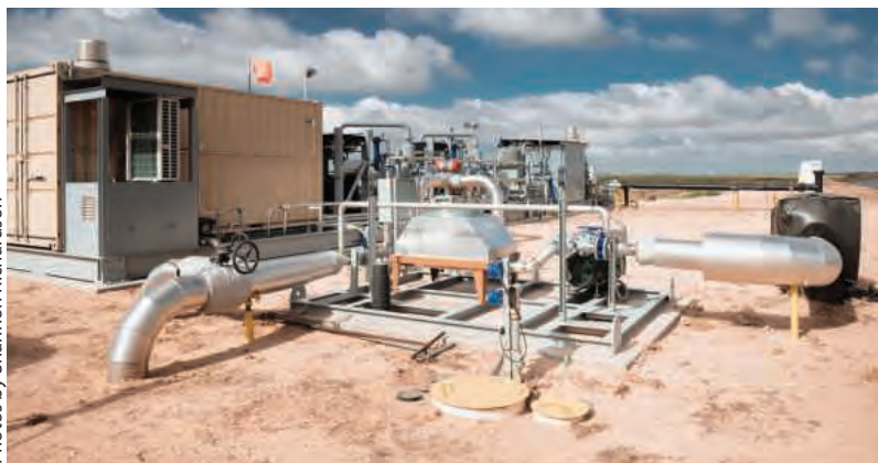
Full Circle Jerseys' methane digester near Dalhart, Texas, includes a biogas inlet blower, control room and Roeslein membrane upgrading system.
