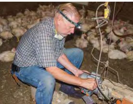
Calvin Becker replaces a feed-line motor in a broiler house.
